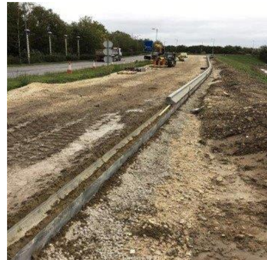
Swale drainage works adjacent to the new slip road
